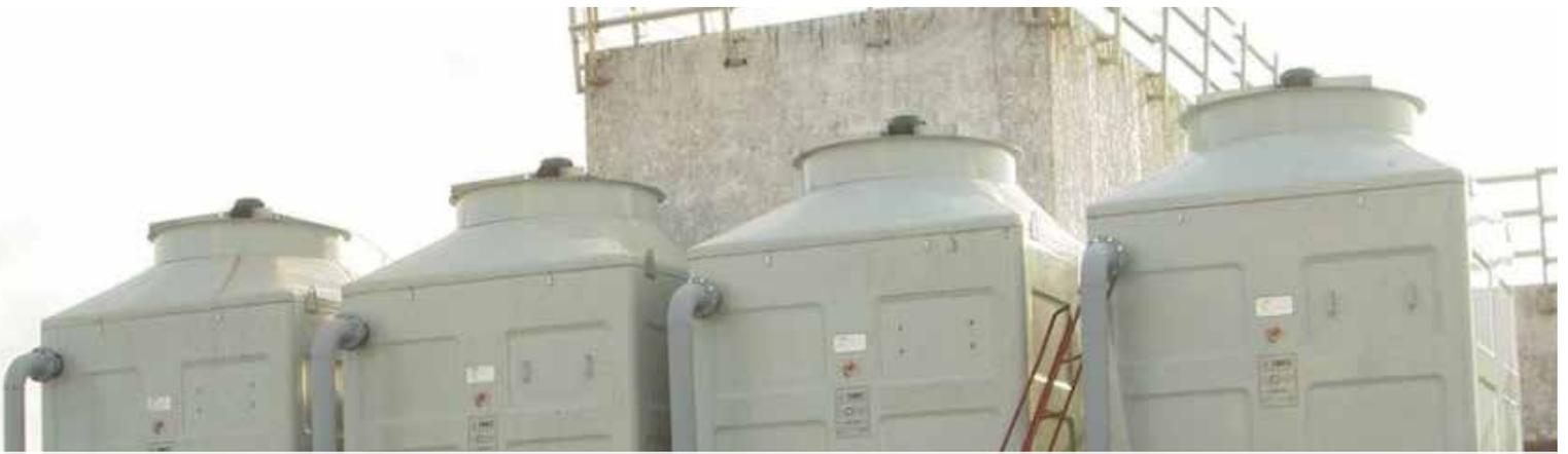
Our package range of towers namely the FGS and the FM towers are manufactured in our works and transported to site complete and ready for installation.
